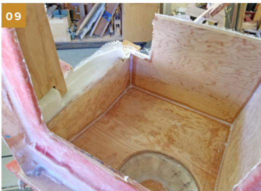
Filleting the back side of the plywood stiffeners.
