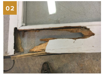
02 The rotted wood has been removed.
