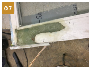
07 The epoxy cured and the mold was removed. Exterior view.
