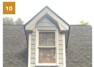
10 Reinstalled exterior view.
