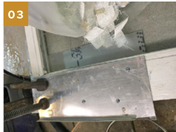
03 The mold piece was screwed and clamped in place.
