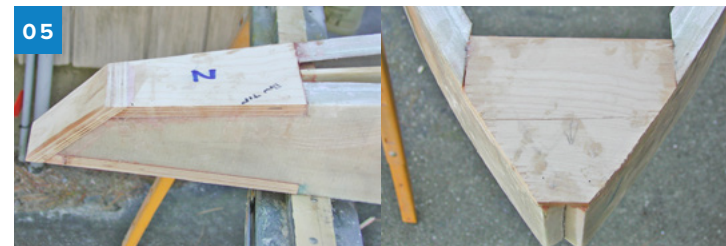
05 Stem blocks were installed to allow for the assembly of bulkheads, decks, etc. at a future time.
