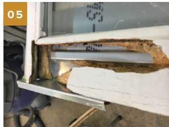
05 An exterior view of the taped mold piece.
