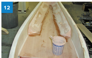
The stiffeners were epoxied in place with 105/206/403.
