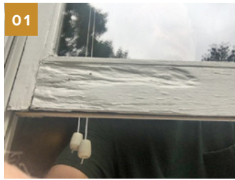
01 The bottom member before beginning the repair.
