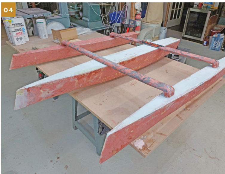
The shaped foam was covered with two layers of 4 oz. fiberglass.
