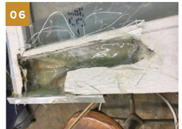
06 Wet-out pieces of fiberglass cloth were placed into the damaged area.
