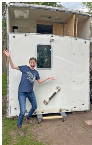
The rear wall has been removed from the camper.
