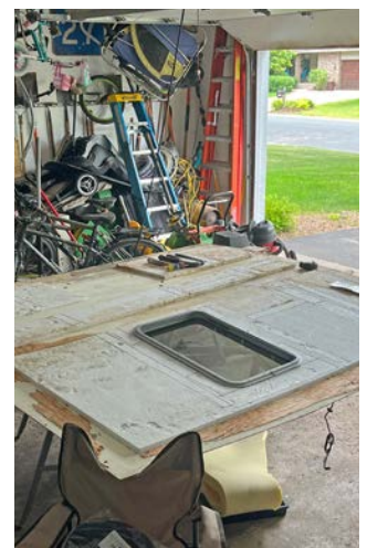
The panel has been relocated to the workshop to begin demolition.
