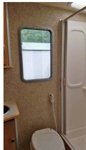
Finished wall from the inside (above) and outside (below).
