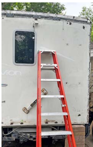
The back of the camper with all exterior trim removed.
