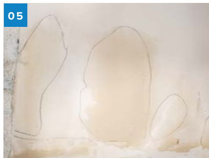
05 Mark the low areas and then remove the pencil lines with sandpaper, so that the thickened epoxy will bond well to the surface.
