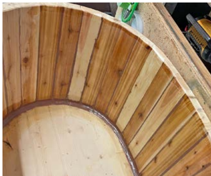
Fiberglass tape was applied to the fillet around the base and 4 oz fiberglass fabric to the interior walls.
