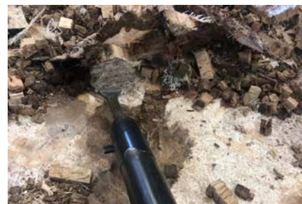
Removing the rotted balsa with a pneumatic chisel.
