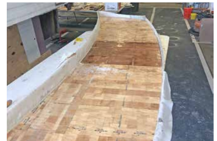
Release fabric is installed over the new balsa.
