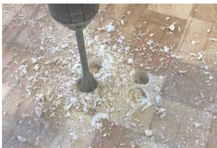
Oversizing holes for the thickened epoxy.
