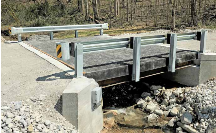
IACMI FRP Composite Bridge
