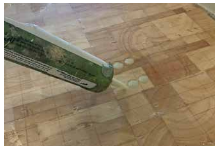
Applying thickened epoxy with an 810 Fillable Caulking Tube.
