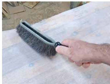
The sanded transom was then brushed clean and wiped down with alcohol and a paper towel.
