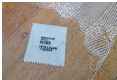
The transom is roughly 9 sq.ft. To adhere the veneer, I chose 105/207 in case there was bleed-through onto the veneer. I mixed two batches of five pump strokes each, and five teaspoons of 403 Microfibers Adhesive Filler. This made a honey-like consistency. I spread this mixture on with a notched trowel.
