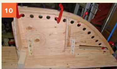
Internal stem mounted on bow stem mold.
