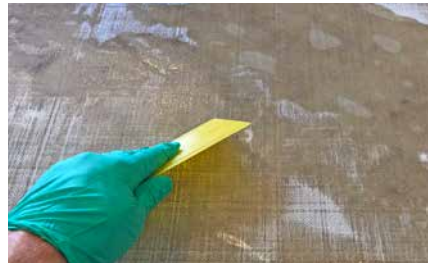
Wetting out fiberglass with epoxy.
