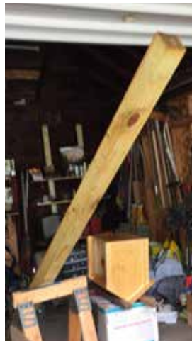
Far Left: The natural wood of the library. The roof has been removed for easier application of the epoxy. Left: The library and the post have both had multiple coats of epoxy applied to protect the wood from moisture. Right: The epoxy stabilizes the wood's moisture content providing for a more stable base for the exterior paint. Far Right: The post is set in an annulus of concrete to counteract the weight of the library once it is filled with books.
