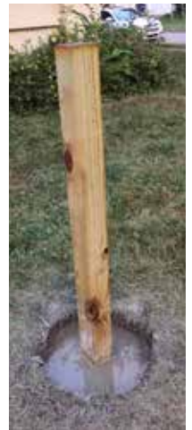
Far Left: The natural wood of the library. The roof has been removed for easier application of the epoxy. Left: The library and the post have both had multiple coats of epoxy applied to protect the wood from moisture. Right: The epoxy stabilizes the wood's moisture content providing for a more stable base for the exterior paint. Far Right: The post is set in an annulus of concrete to counteract the weight of the library once it is filled with books.
