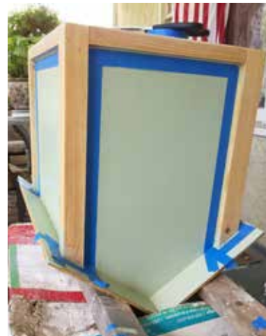
Far Left: The natural wood of the library. The roof has been removed for easier application of the epoxy. Left: The library and the post have both had multiple coats of epoxy applied to protect the wood from moisture. Right: The epoxy stabilizes the wood's moisture content providing for a more stable base for the exterior paint. Far Right: The post is set in an annulus of concrete to counteract the weight of the library once it is filled with books.
