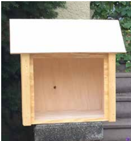
Far Left: The natural wood of the library. The roof has been removed for easier application of the epoxy. Left: The library and the post have both had multiple coats of epoxy applied to protect the wood from moisture. Right: The epoxy stabilizes the wood's moisture content providing for a more stable base for the exterior paint. Far Right: The post is set in an annulus of concrete to counteract the weight of the library once it is filled with books.
