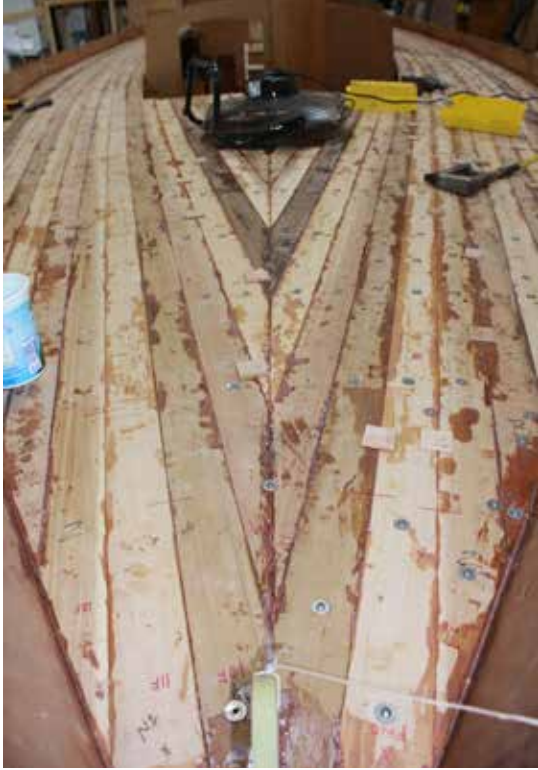
Cabin top planking epoxied in place.
