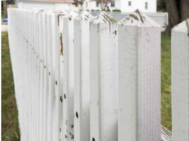
The pickets were cut with a pyramid point on top to minimize the absorption of moisture.
