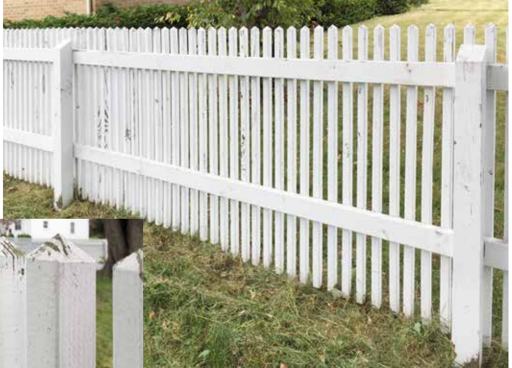
The pickets were cut with a pyramid point on top to minimize the absorption of moisture.
