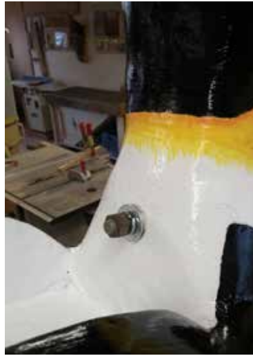
The embedded bolt for attaching the mailbox.
