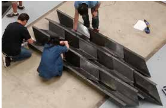
The panels are being assembled into columns.
