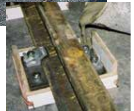
Epoxy grout is being poured into the wooden frame.
