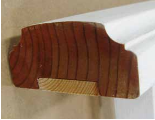
The handrail with end grain coated.
