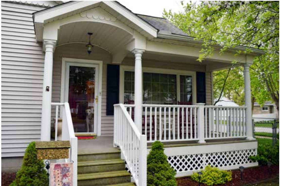
The railing after 15 years...and still going strong.
