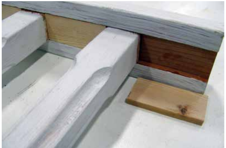
Small wood fill pieces were placed between the spindles to maintain even spacing.
