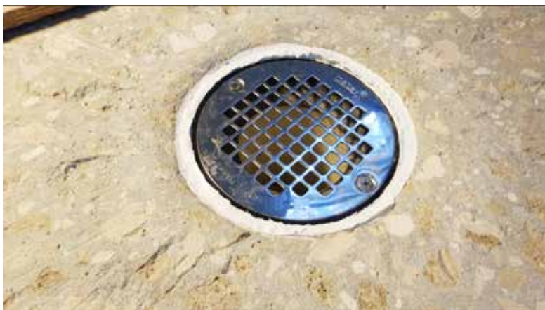
The finished drain installed.
