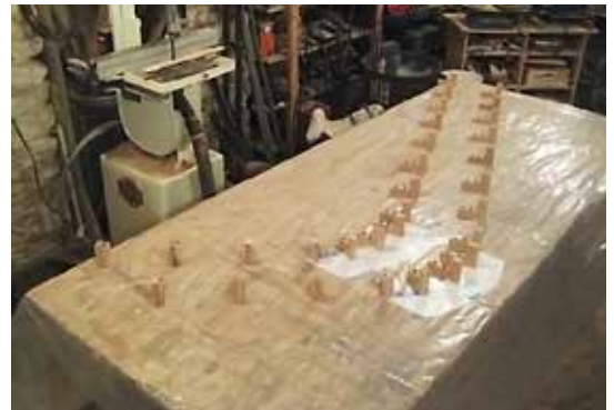
The cranes' legs lofted onto a plywood workbench with poly sheeting and brackets for clamping the laminates.
