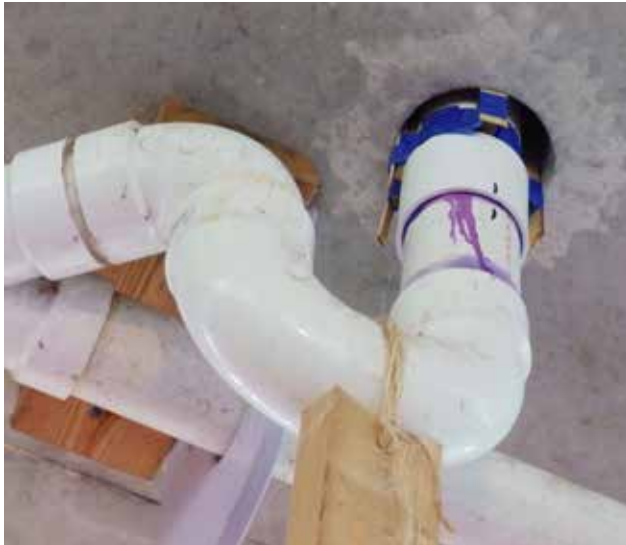
The drain pipe shimmed and centered in place.
