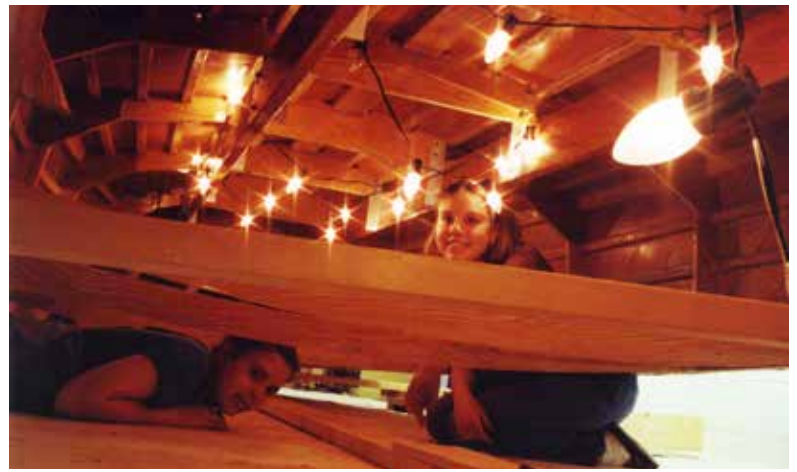
Mark's kids show off the incandescent Christmas lights they strung inside the hull to help make it easier to see the epoxy squeeze out.
