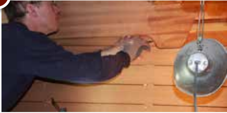
Dave Snyder fitting the ceiling boards on the interior.
