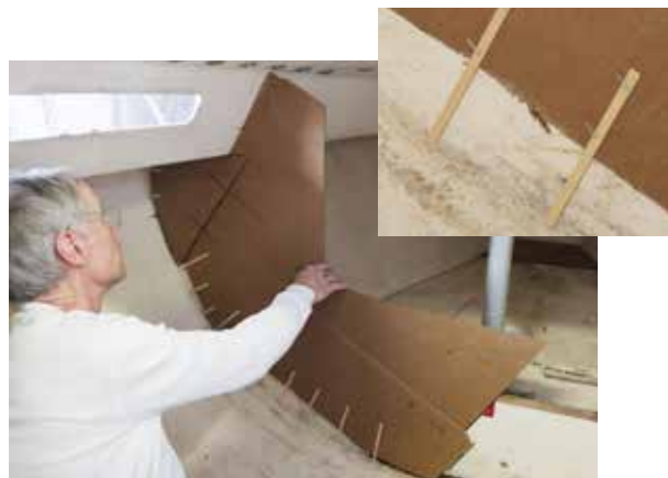
Tom double checking the fit of his template. The inset shows the wooden strips measuring the hull.
