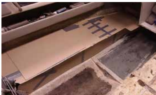
Cardboard templates made for the new plywood sole and stringers
