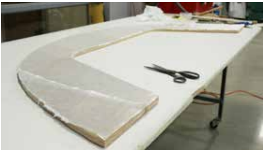
New bulkhead with a layer of 6 oz. fiberglass cut to size
