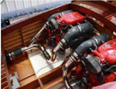
The neat installation of the engines and the shop-made exhaust pipes. The area under the engines is isolated, covered with 6 oz. cloth and WEST SYSTEM Epoxy, then painted white.
