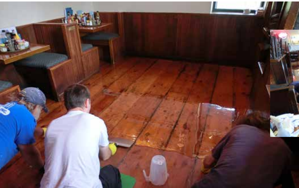
Epoxyworks reader Ted sent us these photos of the floor he installed with 105/207 at a restaurant in Ann Arbor, Michigan.
