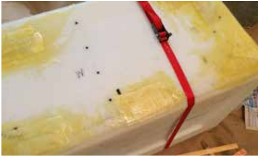
The bottom of the seat shell with cracks filled and reinforced with fiberglass.
