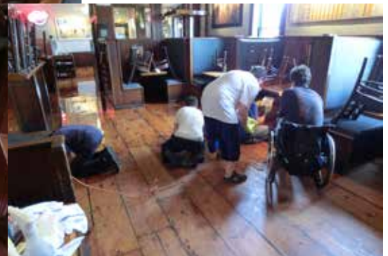
Epoxyworks reader Ted sent us these photos of the floor he installed with 105/207 at a restaurant in Ann Arbor, Michigan.
