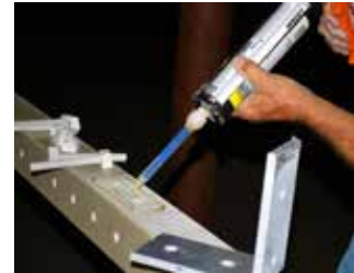
Six10 Adhesive being used to glue bolts and brackets in place
