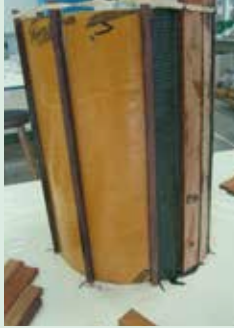
Press strips onto the form forcing epoxy between gaps
