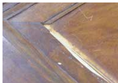
Top left: Damaged door Bottom Left: Close up of damaged section Top Right: New molding cut to size and laying in place Bottom Right: New trim held in place with Six10 and finish nails, the gap being filled with 105/205 with 405 Filleting Blend for color.
