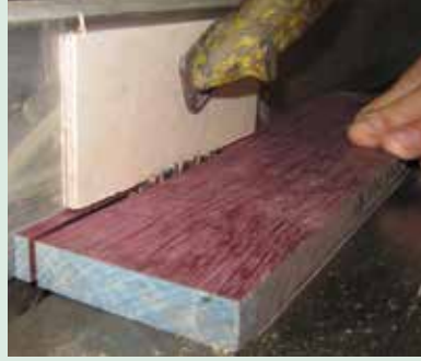
Rip wood strips to cover the form
