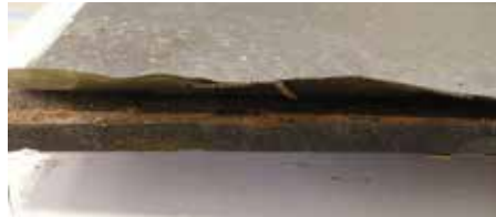
Top: The damaged bottom of the door. Above: The aluminum facing being peeled back
