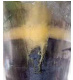
The front of a keel repair in progress. The crack has been cleaned, widened and filled with G/flex 655.
