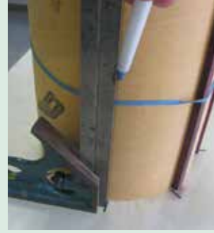
Mark vertical lines for alignment and attach accent pieces
