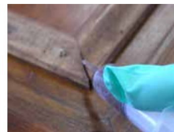
Top left: Damaged door Bottom Left: Close up of damaged section Top Right: New molding cut to size and laying in place Bottom Right: New trim held in place with Six10 and finish nails, the gap being filled with 105/205 with 405 Filleting Blend for color.
