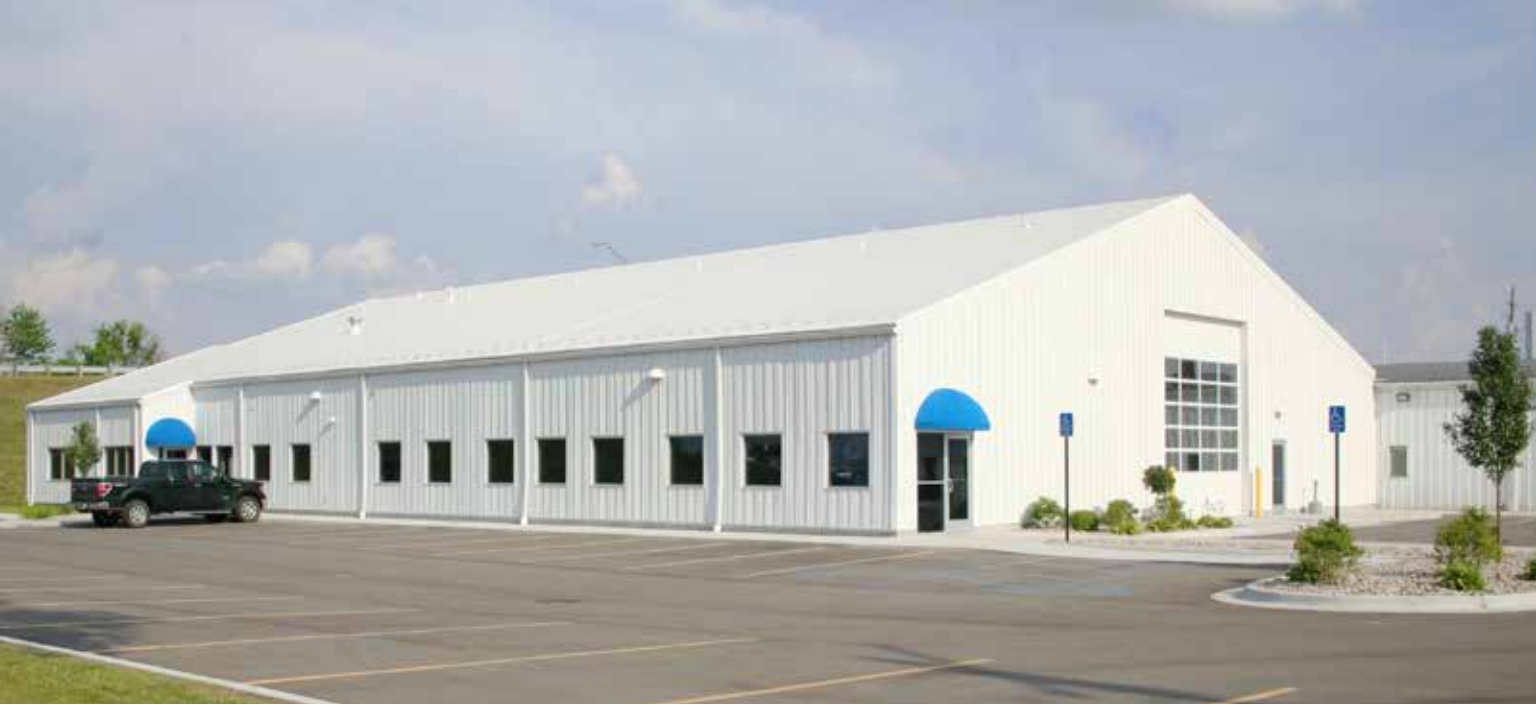
The new technical building
