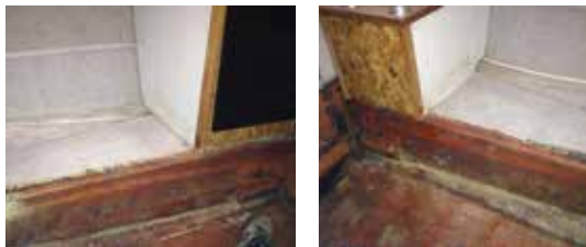
Two views of the cabin with the carpeting removed
