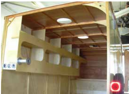
Three 12" diameter holes were cut into the top as skylights made out of polycarbonate.
