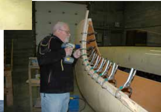
Patently applying the curved end sections
