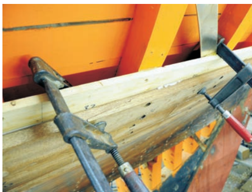
A "nibbed scarf" joint in the outer planking being glued together in place over the inner planking.
