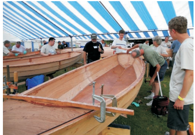
On day three the decks were installed. At the end of the show, the weary families headed home to install the thwarts and seats and get started on the big tasks, sanding and finishing.
