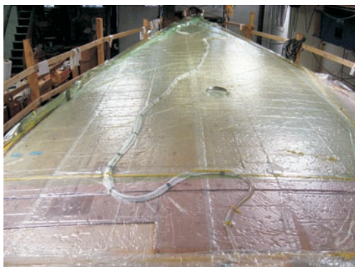
Two layers of 1/4" plywood are vacuum bagged over cedar planking. Note the staggered joints in the plies.
