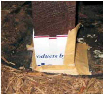
After treating the posts with wood preservative, Blackmon used plastic sign material to make forms around the base of the posts.
