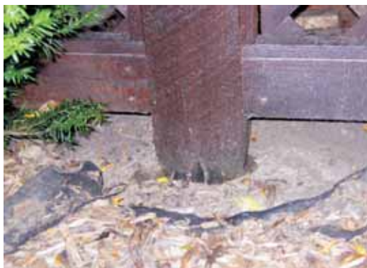
Blackmon's two-story deck is supported by 6×6 redwood posts resting on concrete footings.
