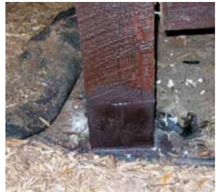
Blackmon finished the repair with a coat of dull brown paint to camouflage the epoxy base.
